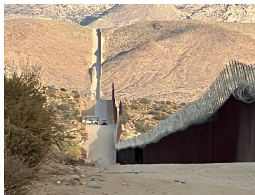
Figure 5. CBP vehicles patrol the only road leading to the Willows site. (Photo from November 14, 2023).
